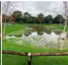
Online SuDS ponds withing localised deepening of detention basins to increase biodiversity
